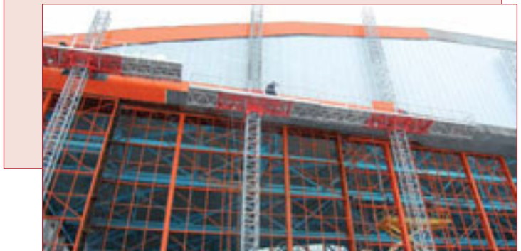
A series of Scanclimber mastclimbers were used to fit the upper cladding and carry out trim work on this building.
