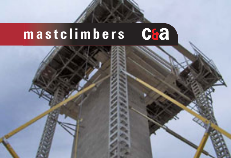
Ultra heavy duty! A four mast Hydromobile M series mast climber installation.
